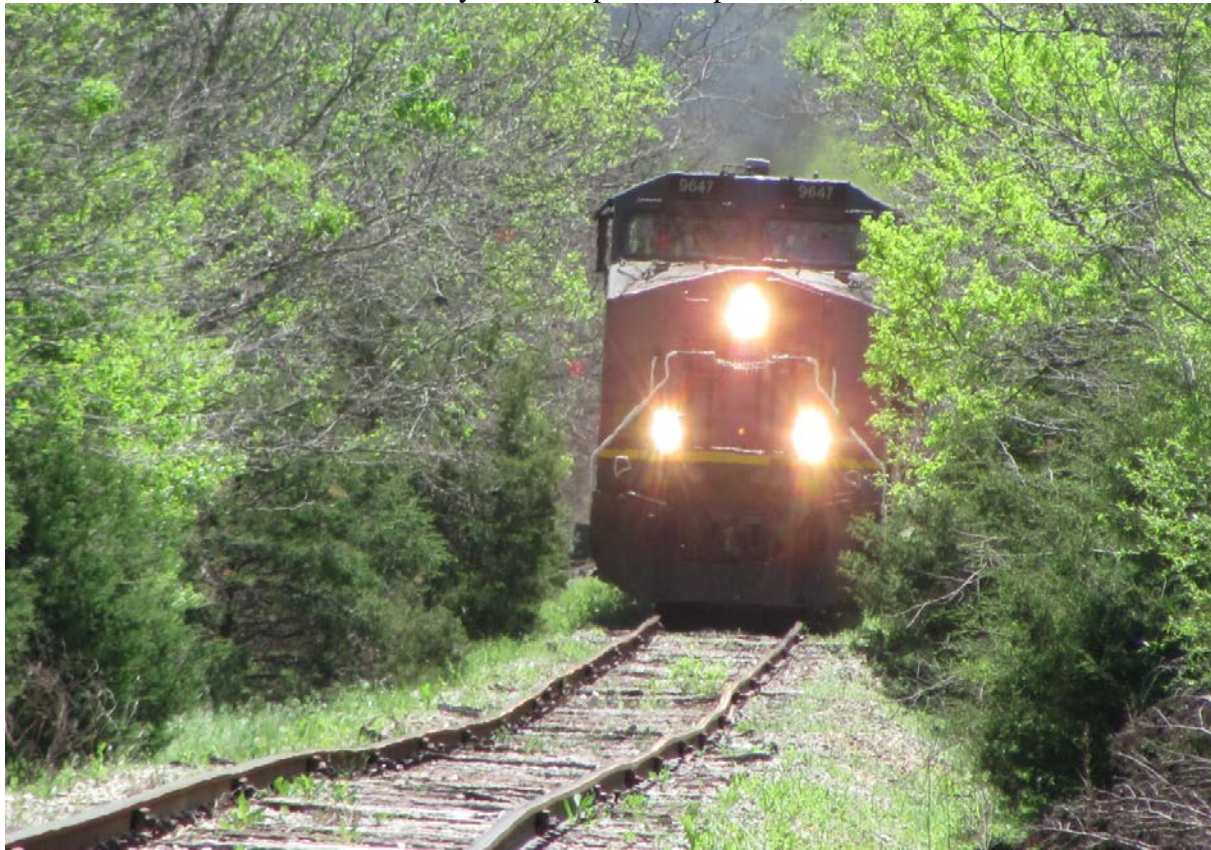
Figure 2 – Deteriorated cross ties, poor rail alignment and profile, and vegetation encroachment on the NETEX/BLR rail line. L. Joyce Davis photo. April 15, 2014.
