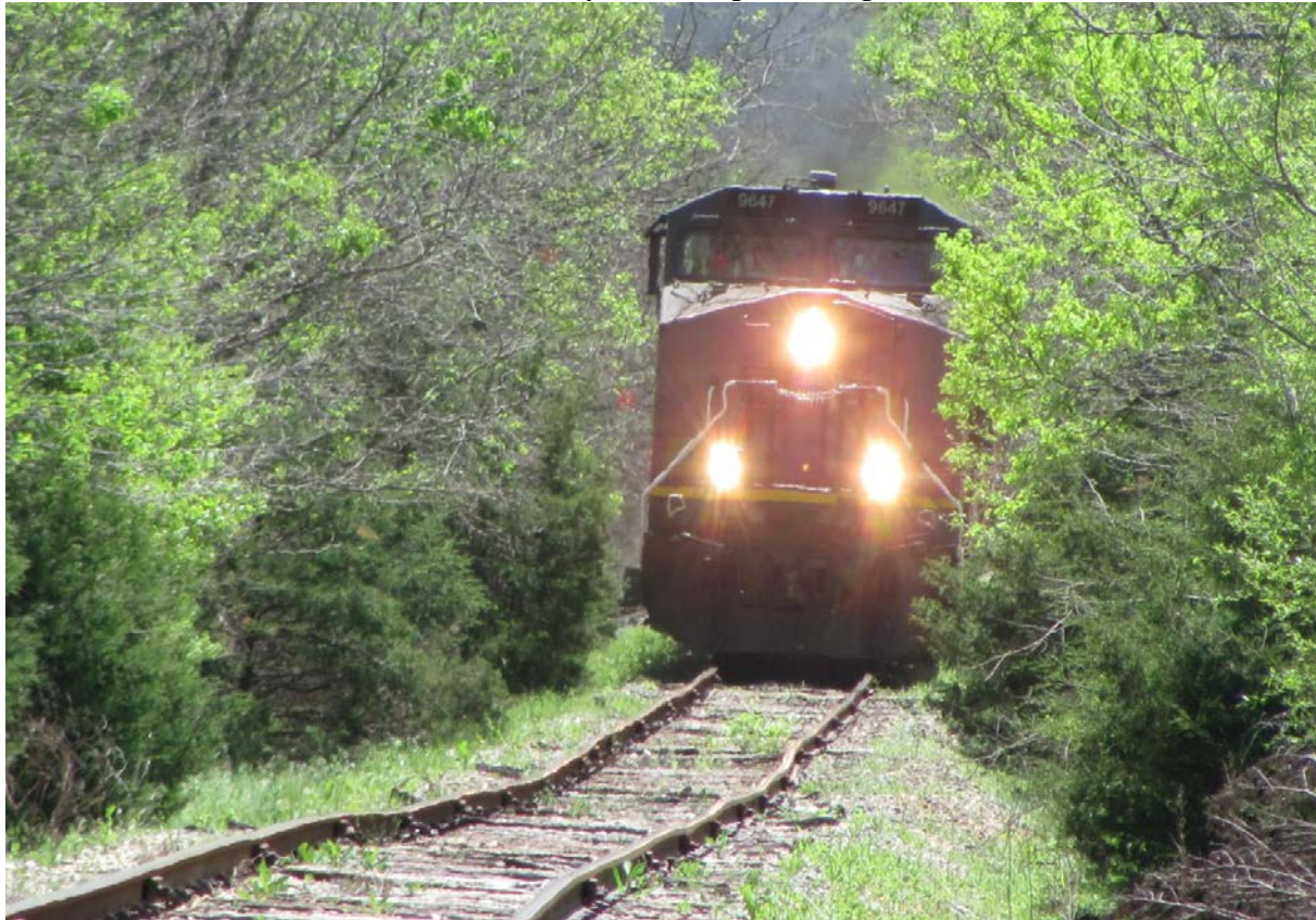
Figure 2 – Deteriorated cross ties, poor rail alignment and profile, and vegetation encroachment on the NETEX/Blacklands rail line. L. Joyce Davis photo. April 15, 2014.
